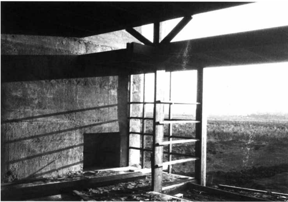
Figure 15 R. M. Schindler. Kings Road House (R. M. Schindler, 1922), West Hollywood, California. Guest studio, 1922. Construction view (Courtesy of the Architecture and Design Collection, University Art Museum, University of California, Santa Barbara).
