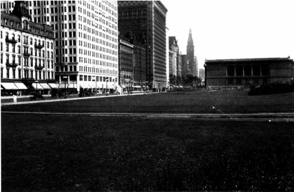
Figure 6 R. M. Schindler. Michigan Avenue and Grant Park, 1915. Art Institute of Chicago (Shepley, Rutan & Coolidge, 1893) is at right (Courtesy of the Architecture and Design Collection, University Art Museum, University of California, Santa Barbara).
